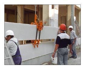
Flat grab FG/U with catch hook for the safe erection of wall panels, to be carried out also high above the ground.
