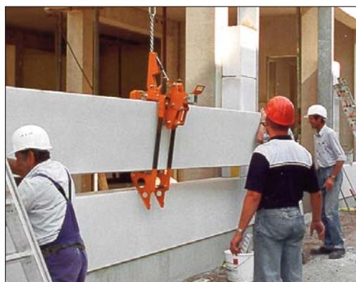
Flat grab FG/U with catch hook for the safe erection of wall panels, to be carried out also high above the ground.
